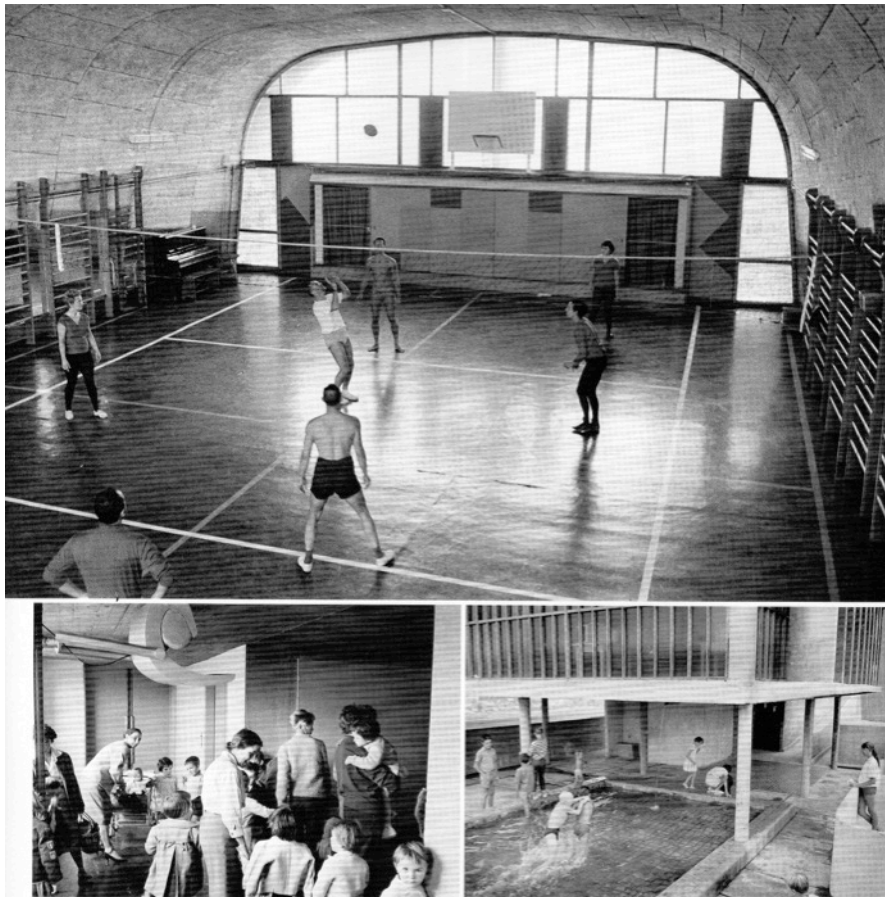
Figure 16. Rooftop gymnasium, pool, and play areas at Unité d'Habitations Marseille. Jean-Louis Cohen and Tim Benton, Le Corbusier Le Grand , (London: Phaidon, 2008), 426.
