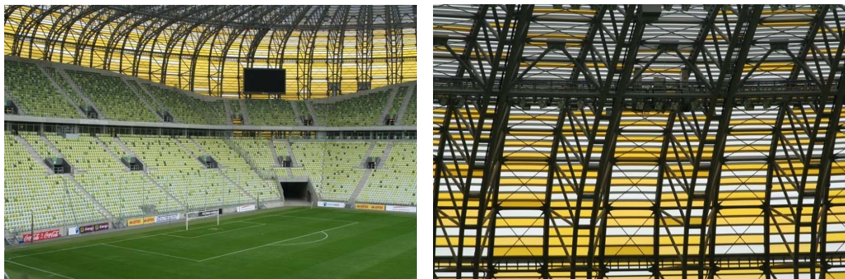
Figure 5, 6. The interior of Enea Arena with the view of stands and girders
