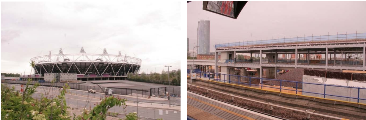
Figure 7, 8. The Olympic Stadium and the suburb of Stratford under renovation
